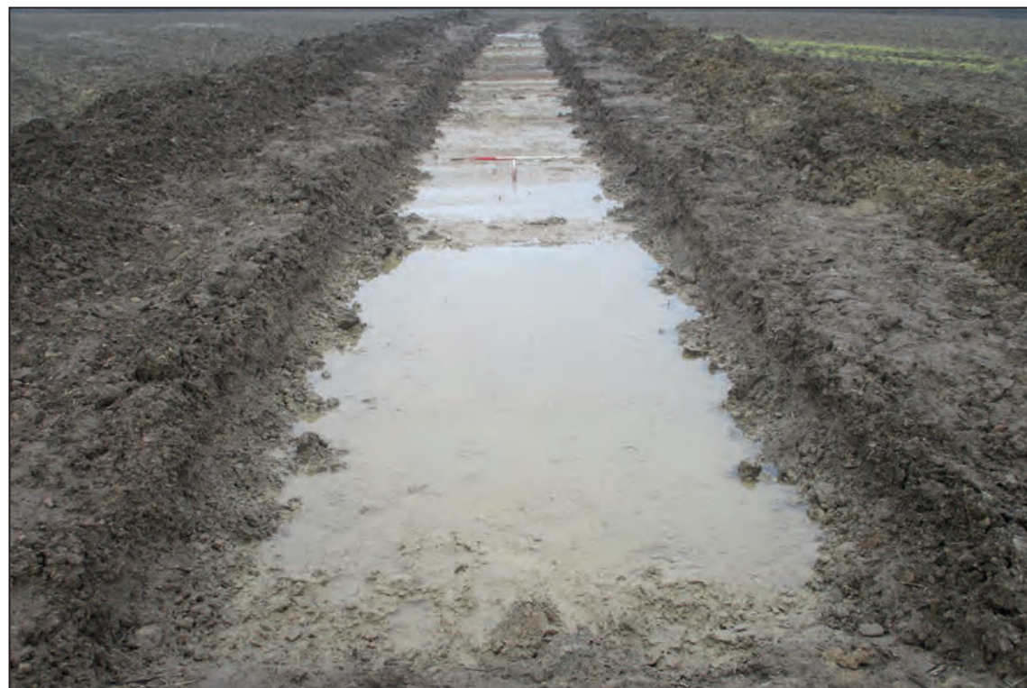
Trench 171, looking north-west (1m scales)
