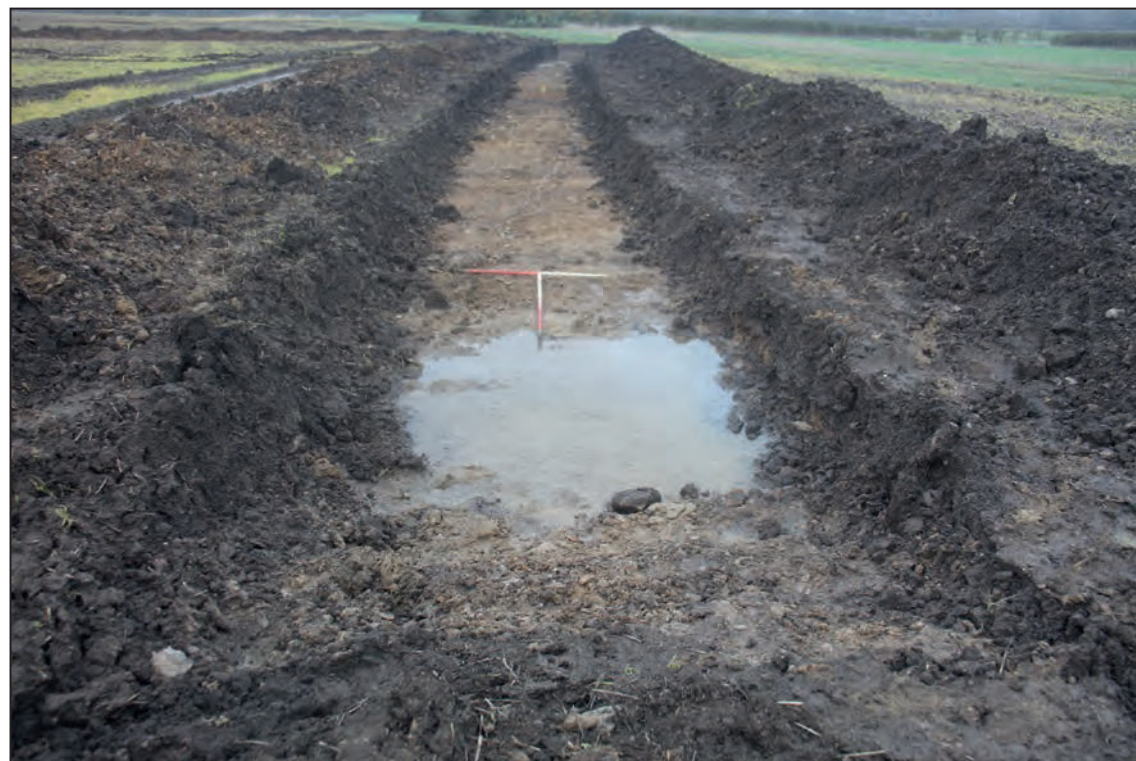
Trench 159, looking west (1m scales)
